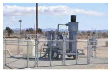
that carry the treated air away from ground level. The cleanup efforts at the former George AFB do not make the air at George dangerous or unhealthy in any way. These SVE systems are working to reduce and eliminate residual soil and groundwater contaminants to ensure the air remains healthy for future generations.
